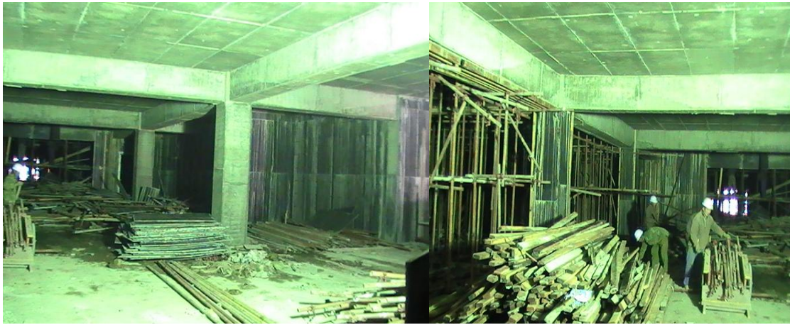
Figure 11. Plastic Construction Templates Can Be Re-Used or Sold to Factory for Recycling
