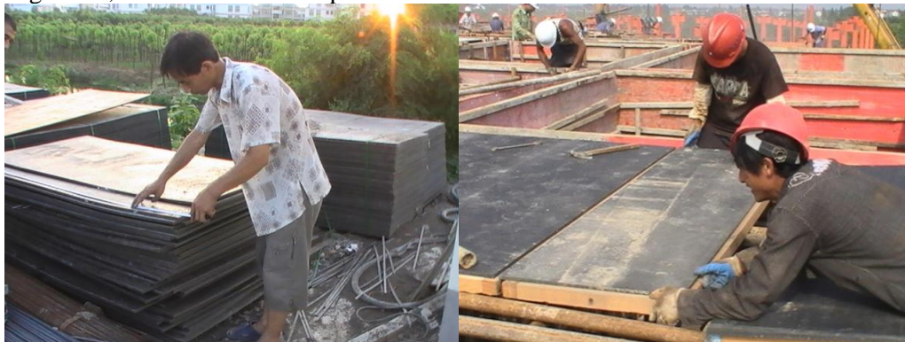
Figure 10. Plastic Construction Templates Are Used to Construct Forms for Poured Concrete
