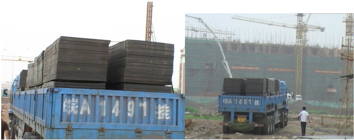
Figure 8. Templates Loaded on Trucks for Delivery
